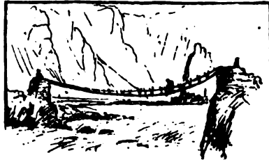
"JHULA" BRIDGE AT KHARTAKSHO.
